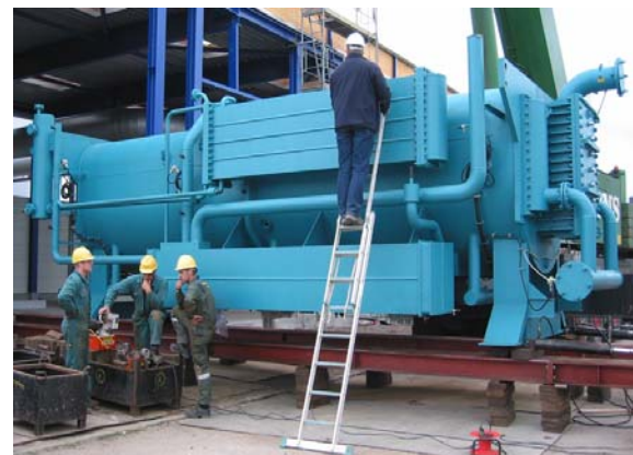
Figure 5: Installation of a heat pump bottom part with common absorber & evaporator vessel.
