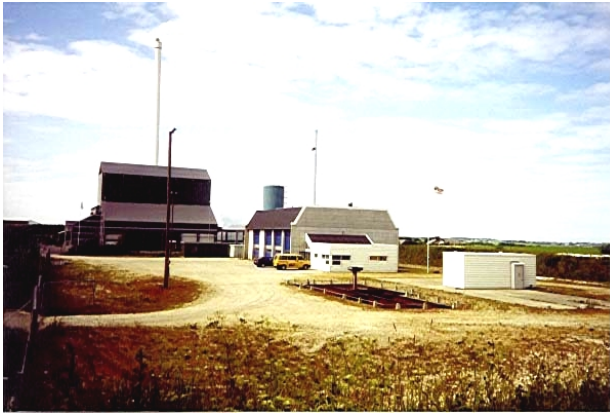
Figure 1. Geothermal plant in Thisted with basin used to remove methane when clean up to sewer, wellhead shelter, geothermal plant, heat accumulation tank and incineration based CHP plant supplying driving heat to the absorption heat pump.
