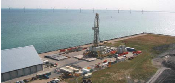
The drilling of the geothermal demonstration plant in Copenhagen.
